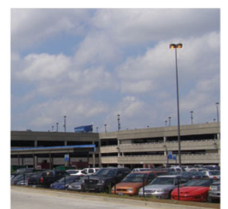
ATL International Airport N. Terminal Parking Deck
